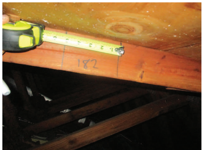
Roof Deck Attachment
