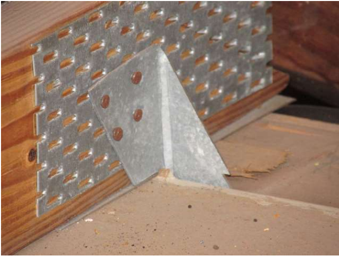
Roof to Wall Attachment
