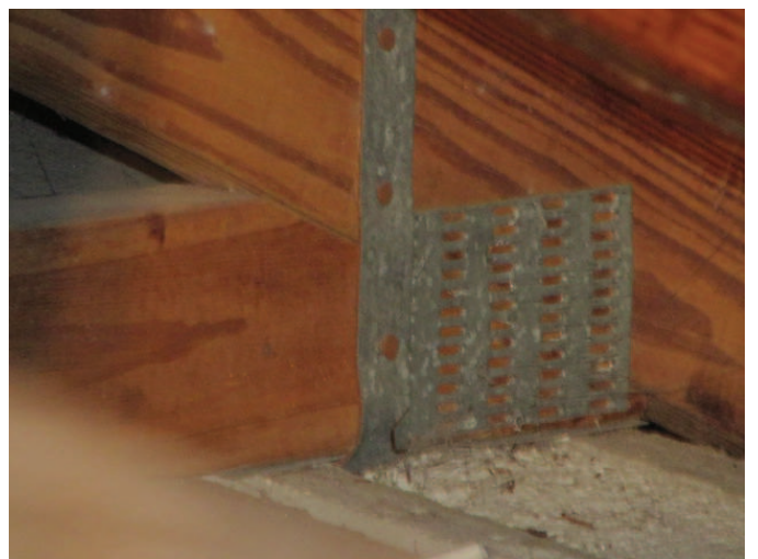
Roof to Wall Attachment
