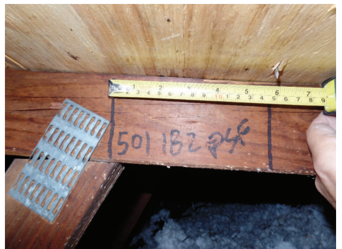
Roof Deck Attachment
