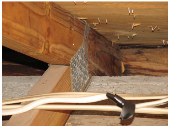
Roof to Wall Attachment
