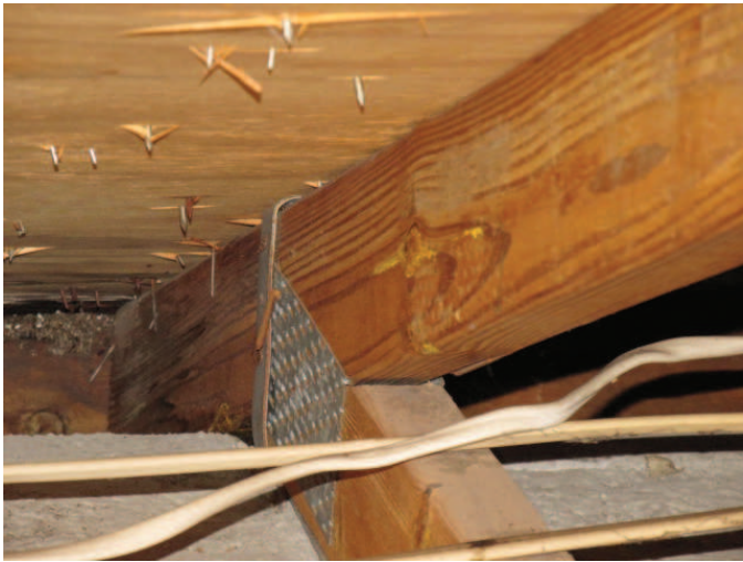
Roof to Wall Attachment
