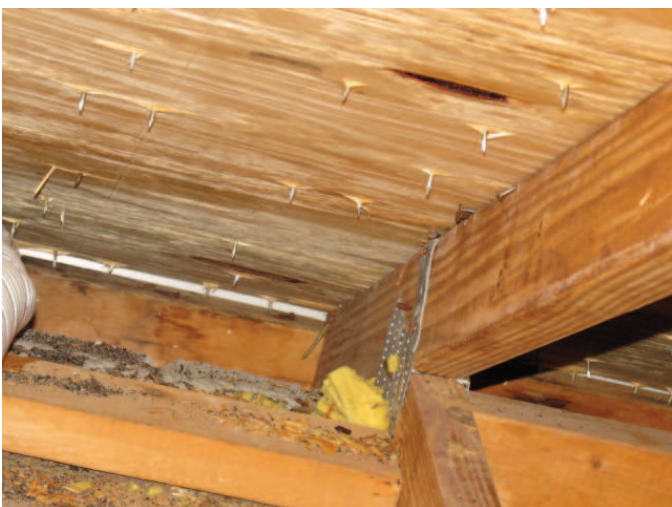
Roof to Wall Attachment
