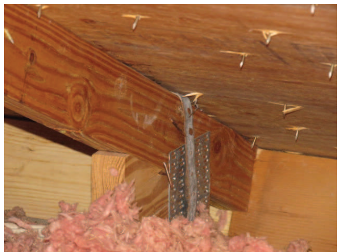
Roof to Wall Attachment
