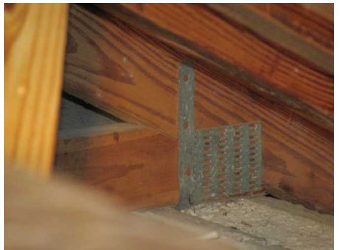
Roof to Wall Attachment
