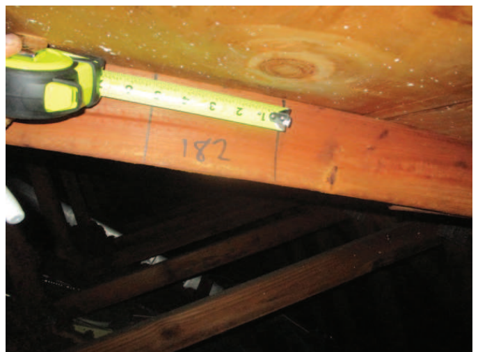
Roof Deck Attachment
