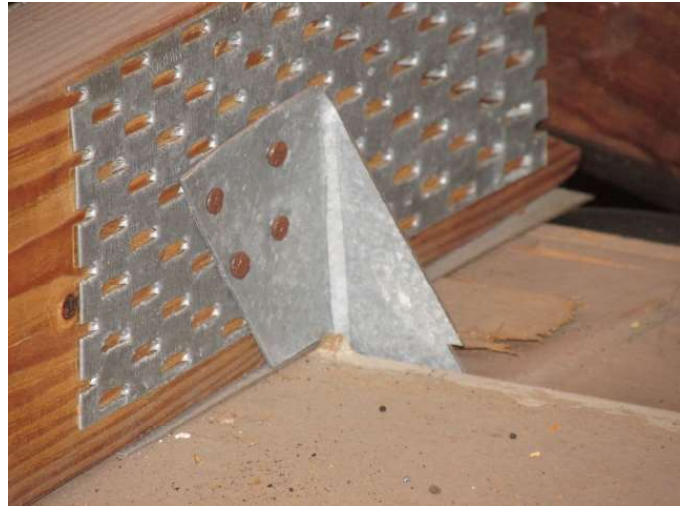
Roof to Wall Attachment
