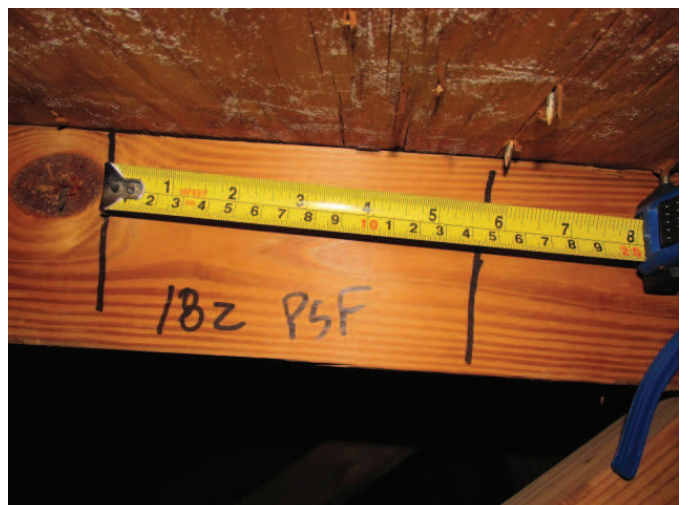
Roof Deck Attachment
