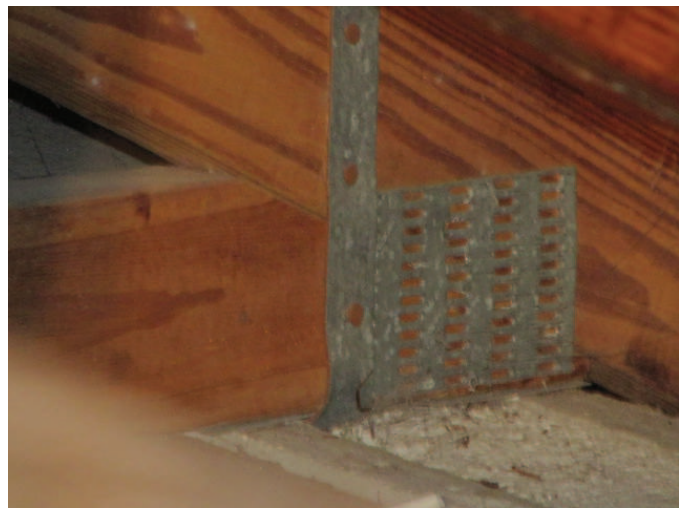
Roof to Wall Attachment
