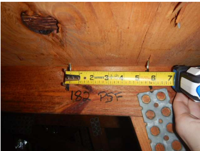
Roof Deck Attachment
