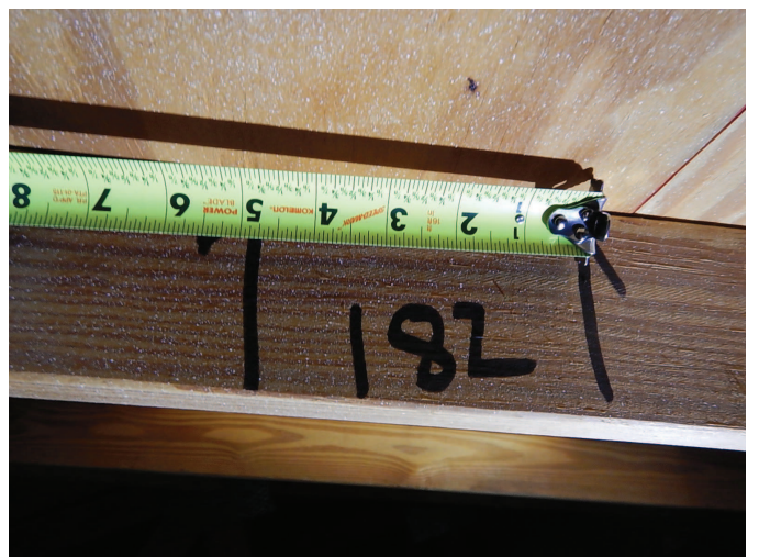
Roof Deck Attachment
