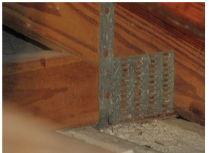
Roof to Wall Attachment
