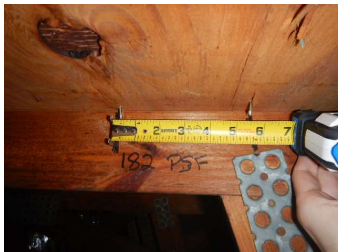
Roof Deck Attachment
