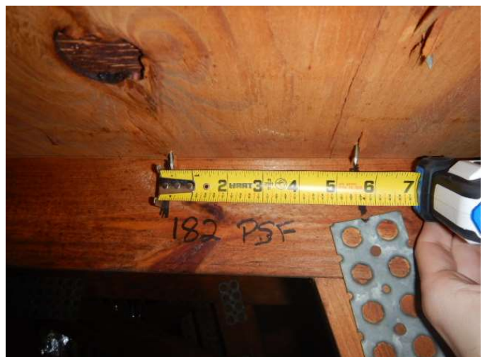
Roof Deck Attachment
