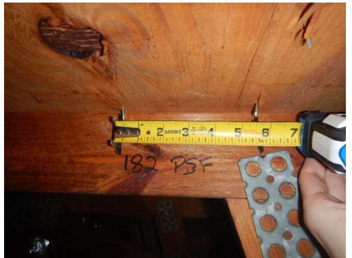
Roof Deck Attachment
