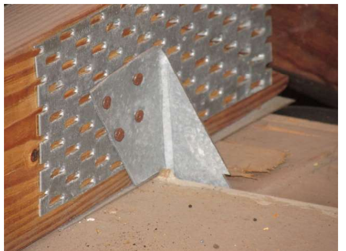
Roof to Wall Attachment
