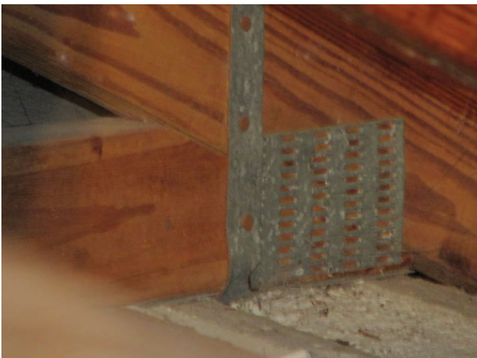
Roof to Wall Attachment
