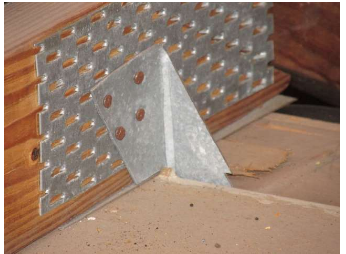
Roof to Wall Attachment
