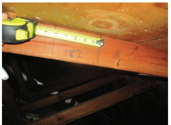
Roof Deck Attachment
