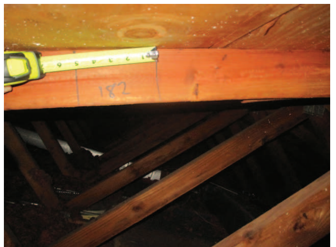
Roof Deck Attachment
