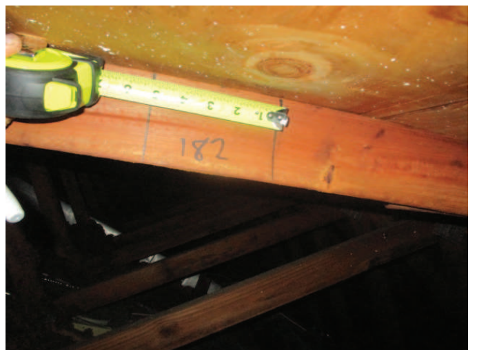
Roof Deck Attachment
