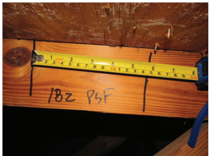
Roof Deck Attachment
