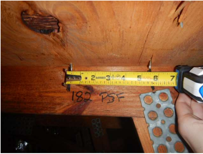
Roof Deck Attachment
