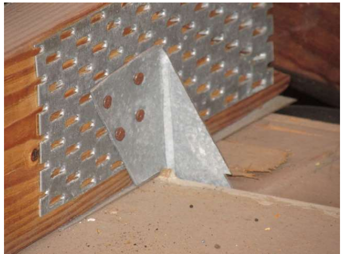
Roof to Wall Attachment
