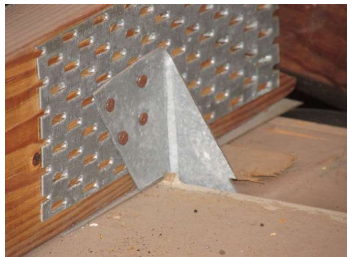
Roof to Wall Attachment
