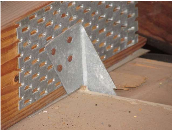
Roof to Wall Attachment
