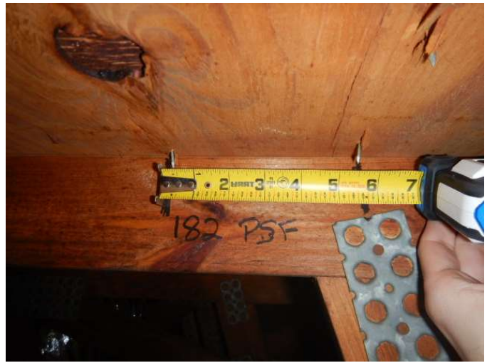
Roof Deck Attachment
