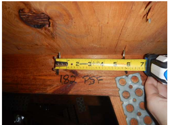
Roof Deck Attachment
